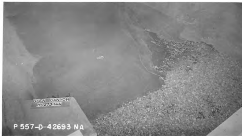
Pre-excavated erosion hole along right bank in powerplant afterbay.
