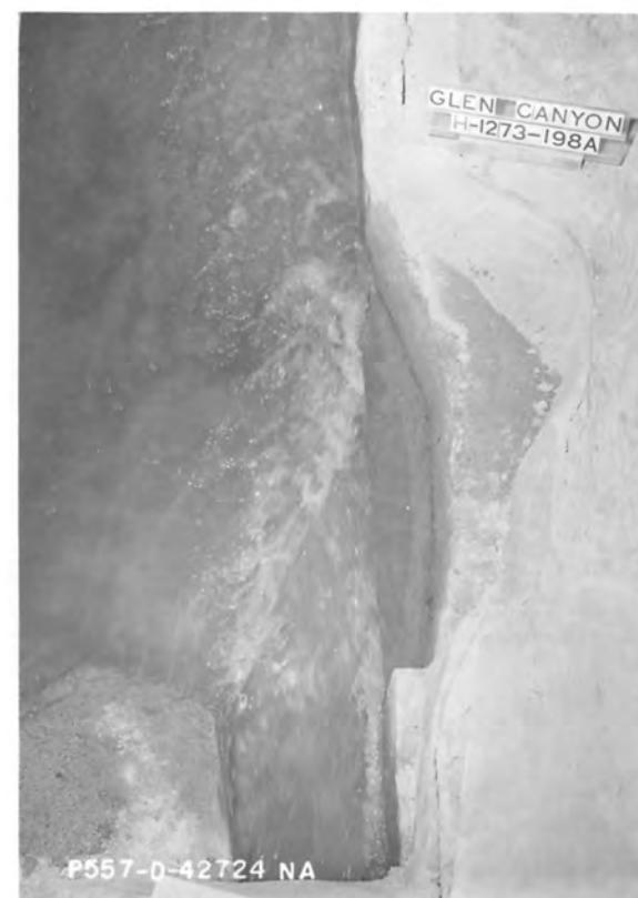
Jet deflected by tailwater surging.
