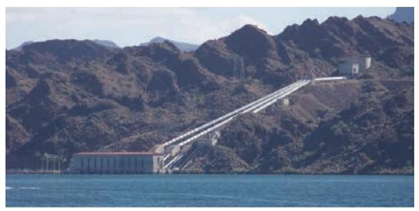
Figure IV-2 Colorado River Aqueduct headworks at Lake Havasu, diverting water from the Colorado River to the Metropolitan Water District of Southern California. Photo credit: Peter W. Culp
