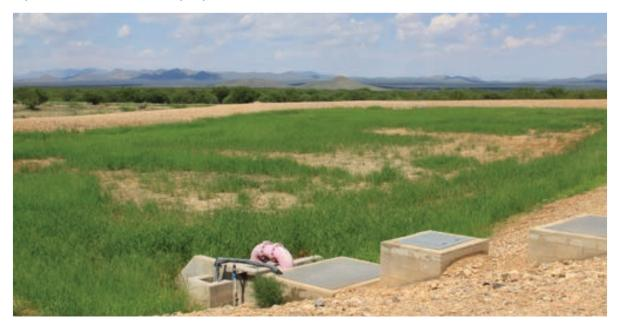
Figure V(C)(2)-2.Groundwater recharge basin near Sierra Vista, AZ. The site is designed to recharge municipal effluent to benefit flow in the threatened San Pedro River. Photo credit: Peter W. Culp
