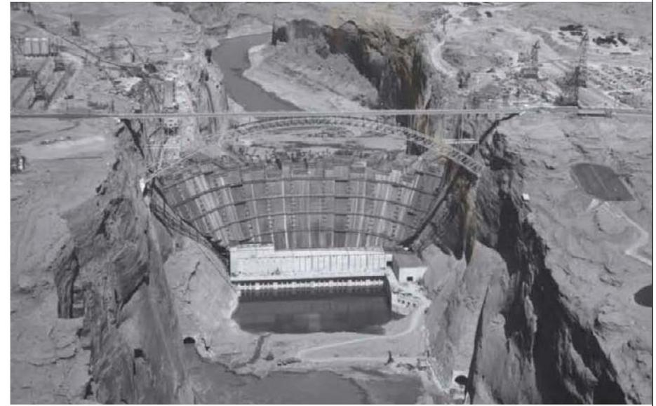
Glen Canyon Dam during construction. Note Colorado River water flowing around the dam at riverbed level through bypass tubes. *Photograph from Bureau of Reclamation.*
