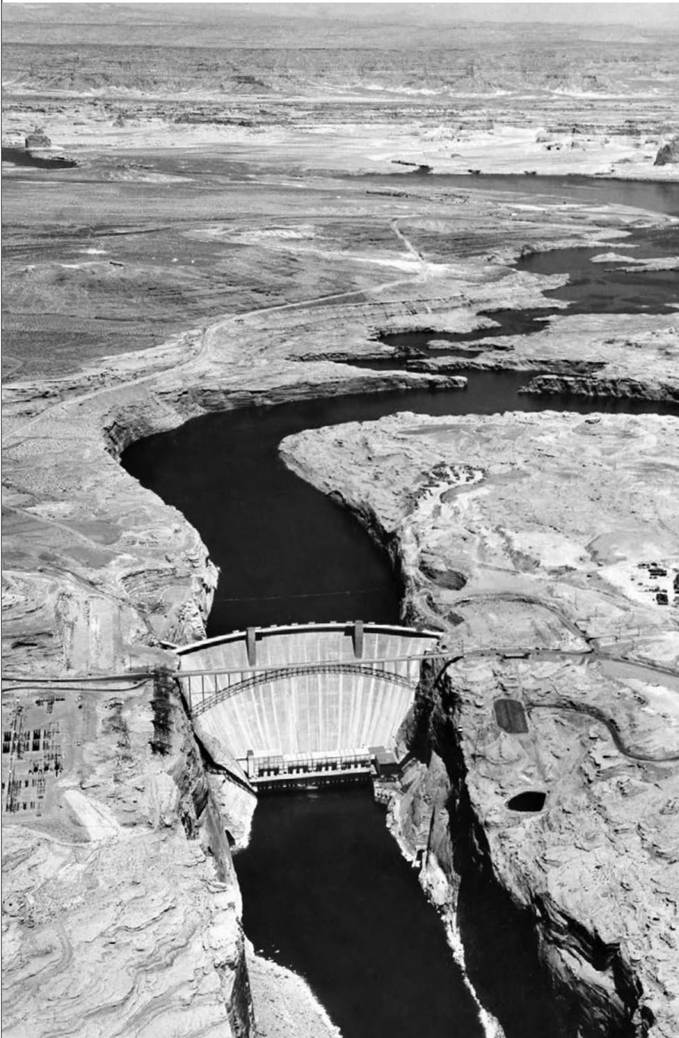
8 Glen Canyon Dam during construction. Note Colorado River water flowing around the dam at riverbed level through bypass tubes. *Photograph from Bureau of Reclamation.*
